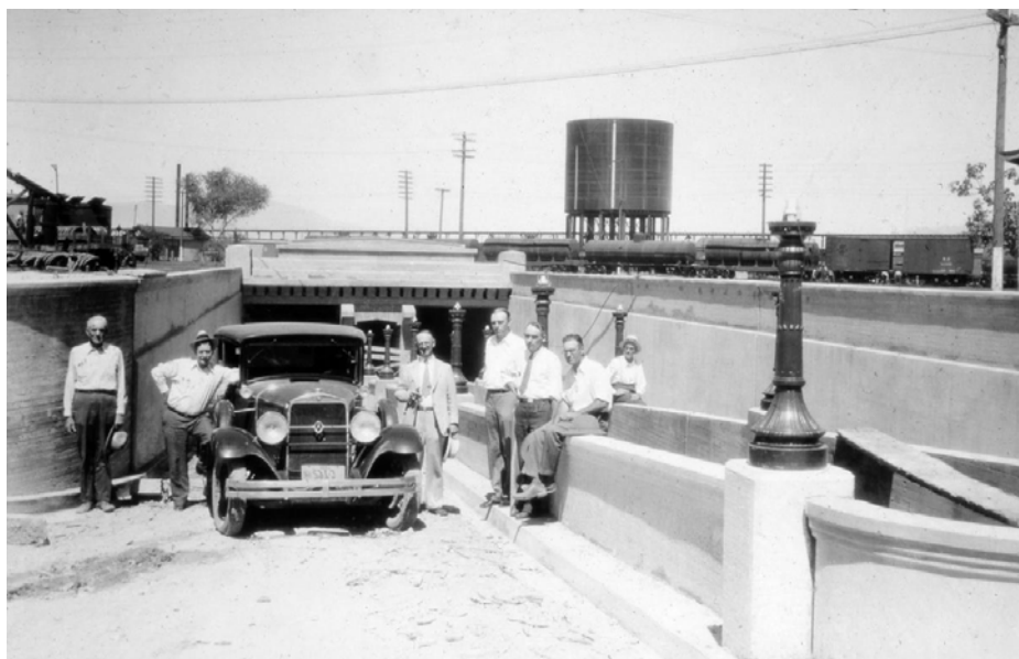
Broadway Road underpass construction in Tucson, ca. 1930s.
